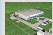
ACCURORMM CENTRAL EUROPE Sp. z o.o. Road w/warszawy (under construction) UL. MINSKA 305A-410 WROCLAW 51-610 POLAND
